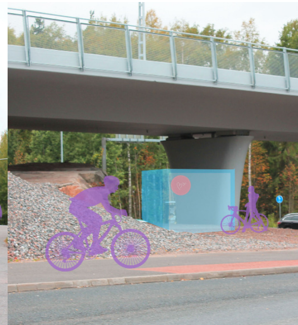
Under a bridge.
