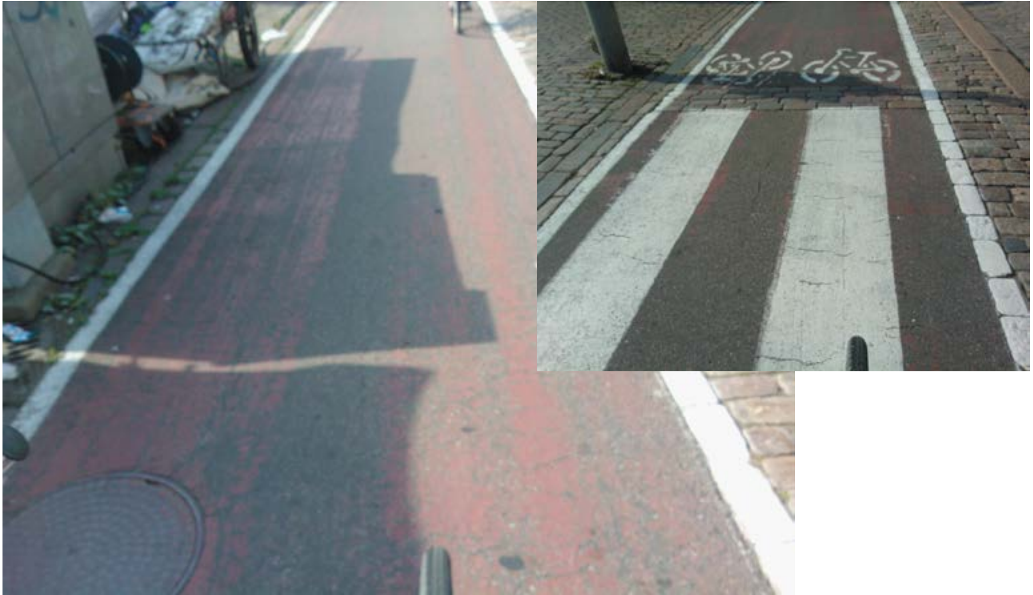
It's good idea to mark the bicycle lane with a different colour but the outcome is poor.
